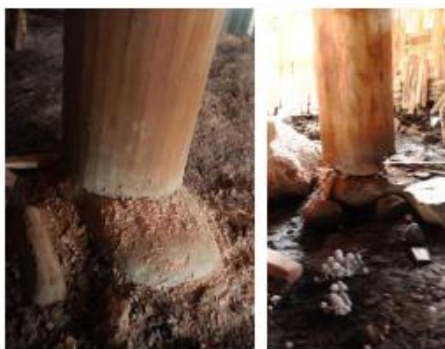
Fig 6. SiPlace the pillars on the stone pedestal directly (left) and the stone pedestal with added stones (right)
